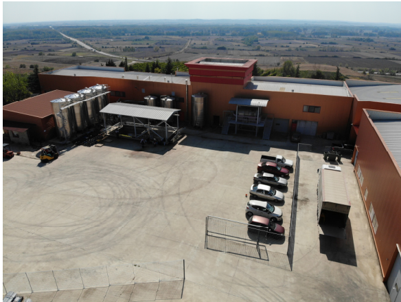
Picture 15. Evritika Kellaria Winery – Building Facilities
