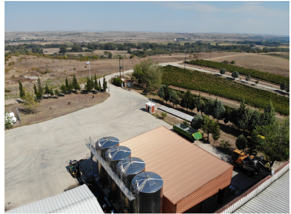
Picture 16. Evritika Kellaria Winery – Building Facilities
