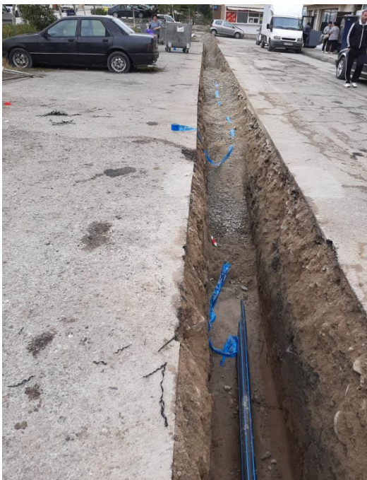
Figure 3.5.3 – Reconstruction of pipeline
