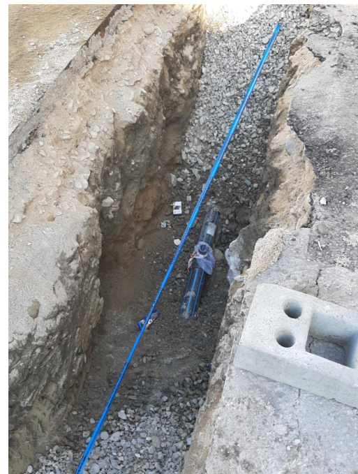
Figure 3.5.4 – Reconstruction of pipeline
