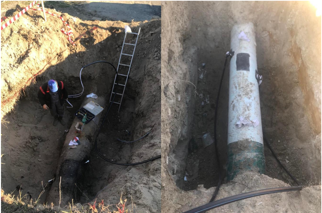
Figure 3.4.2. Installation of the flowmeters
