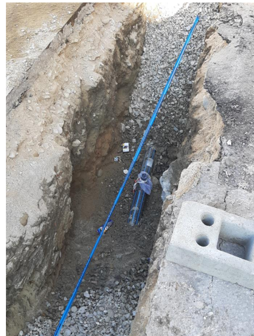
Figure 3.5.4 – Reconstruction of pipeline
