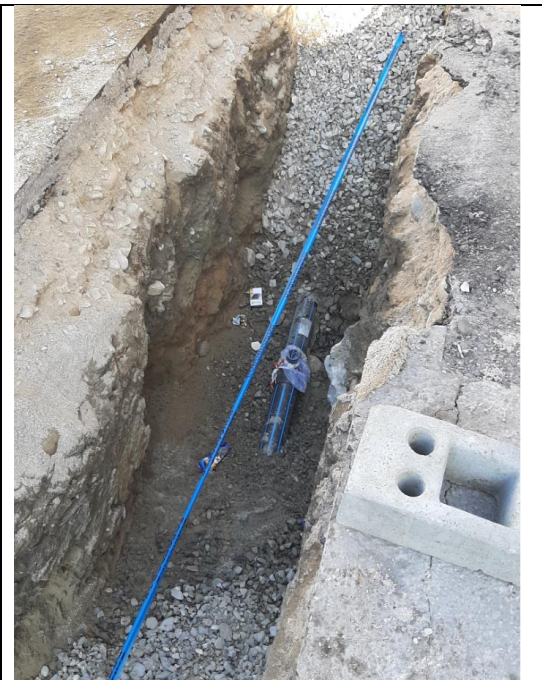
Picture 4 – Reconstruction of pipeline
