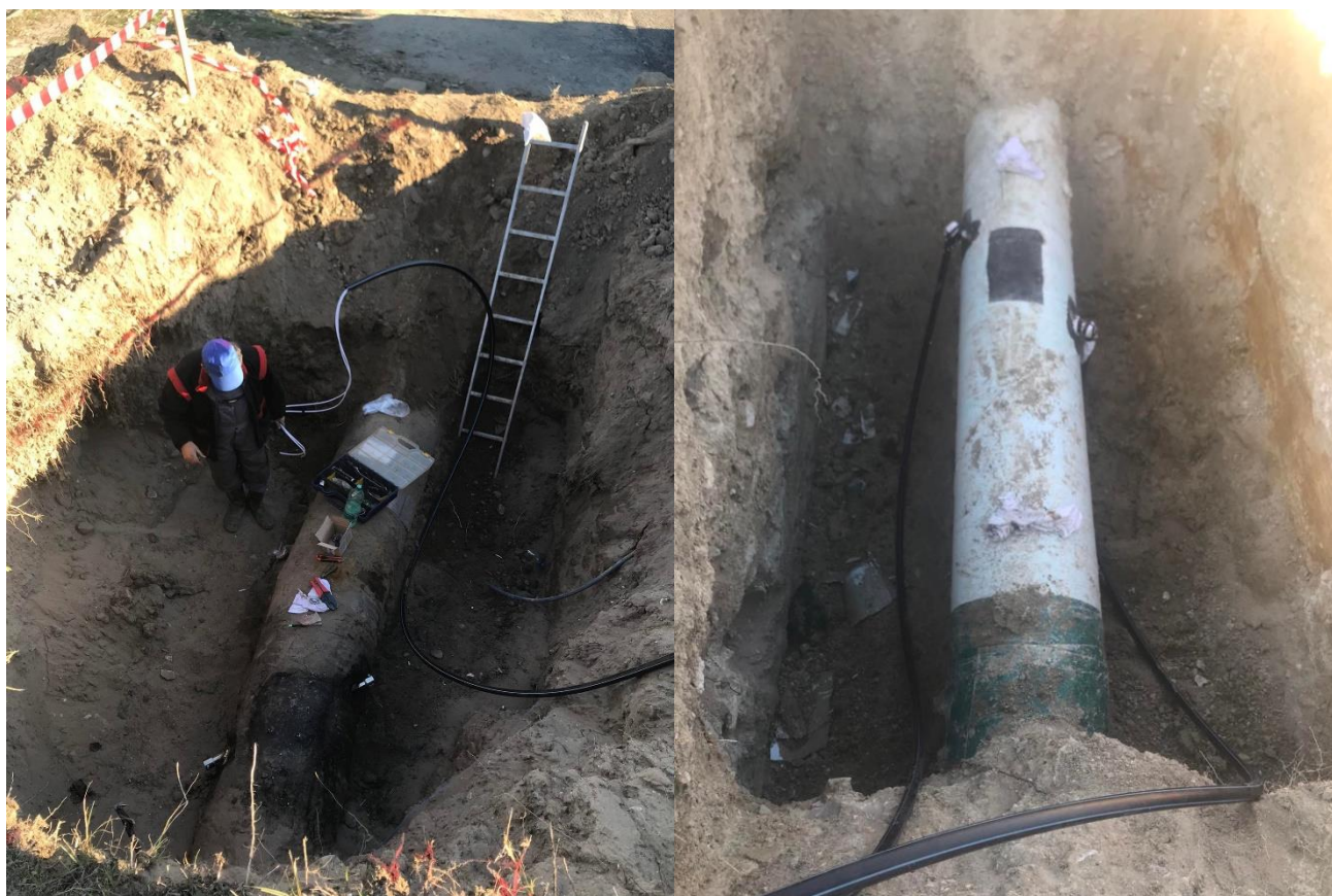
Figure 3.4.4. Installation of the flowmeters
