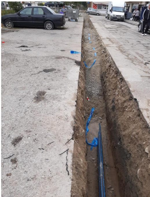
Figure 3.5.3 – Reconstruction of pipeline
