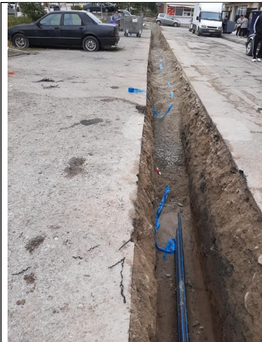
Picture 3 – Reconstruction of pipeline
