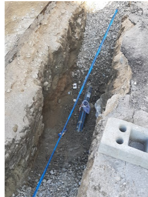
Reconstruction of pipelines
