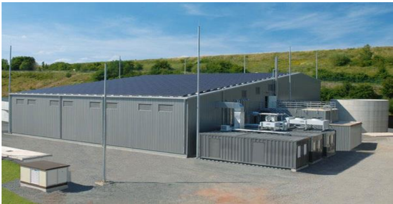
Fig. 11. Dry methanization plant
