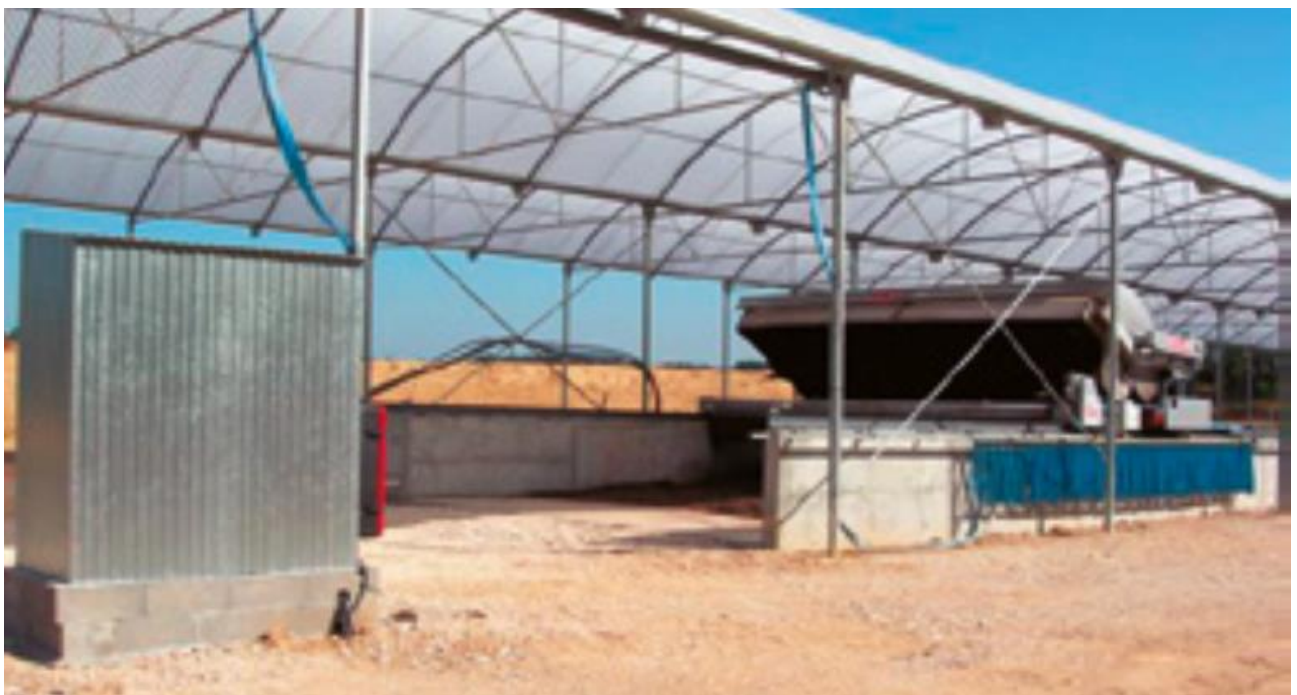
Fig. 7. Composting in open cages with a canopy
