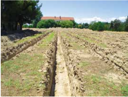
Excavations for the geothermal installation (July 2019)
