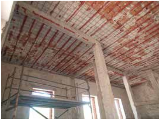
Restoration work in progress (July 2019)
