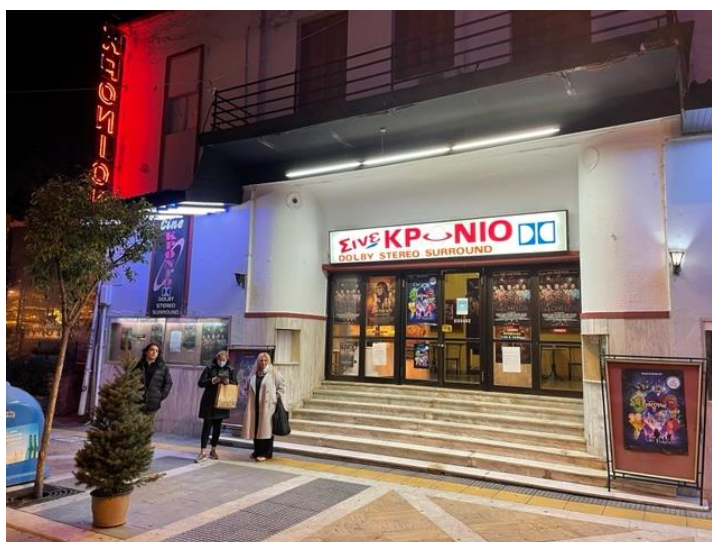
Figure 23. The KRONION Cinema, a listed building together with its open yard, which belongs to the Nursing Home of Serres.
