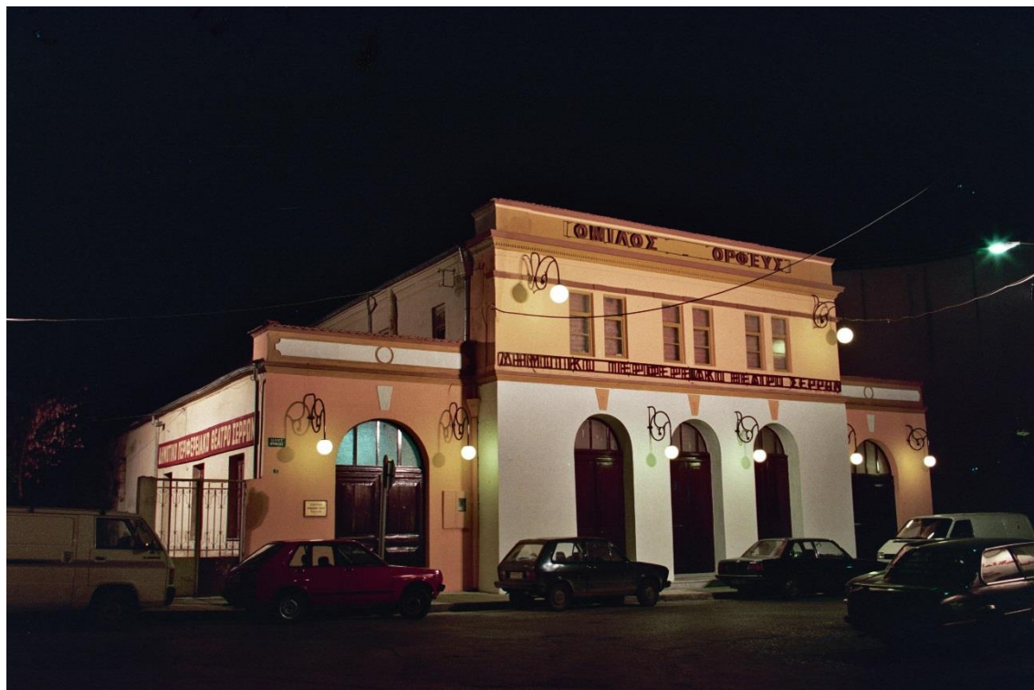
Figure 17. The old ORPHEUS Building.
