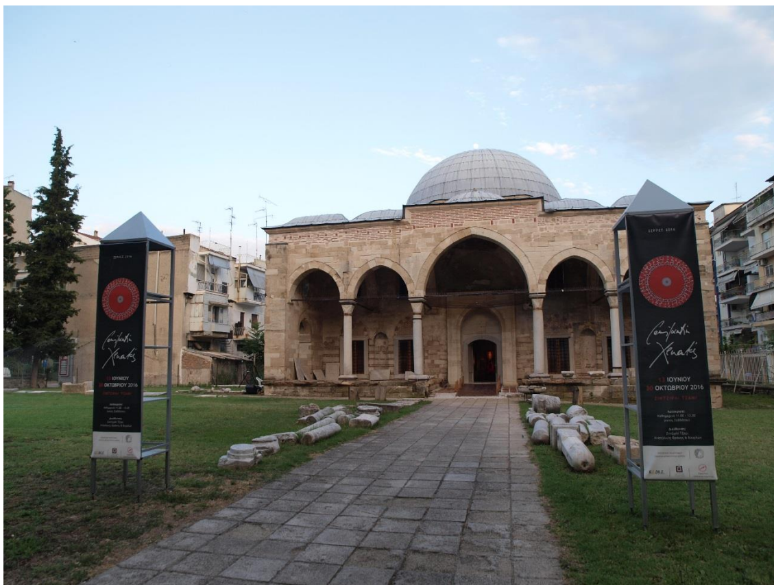
Figure 12. The restored Zincirli Mosque, used as exhibition hall
