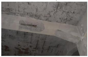
Internal purge of walls with sandblasting
