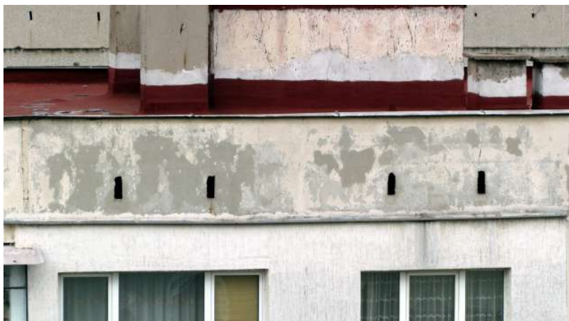
Bats in urban areas often inhabit joints and crevices in buildings
