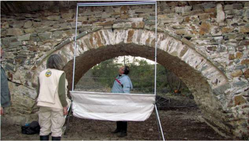
Tuttle Trap placed under bridge
