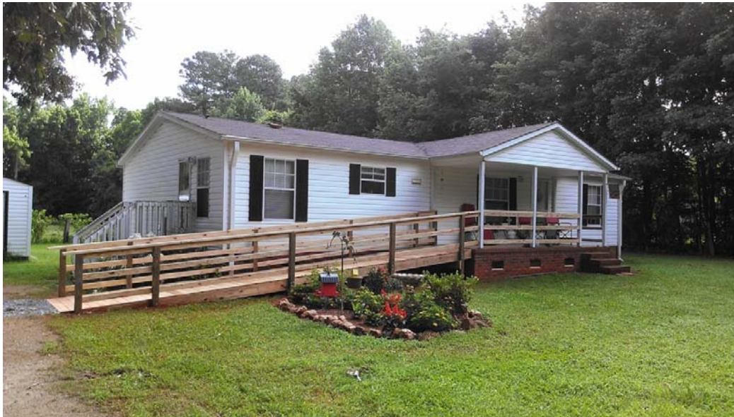
Ramp for improving wheelchair access (Photo: Habitat Cabarrus)
