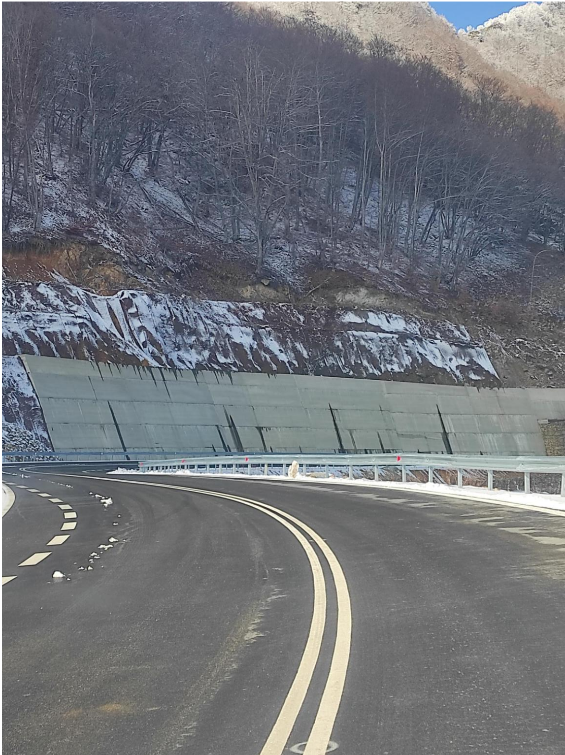
Photo 3: Cut O22 (ch. 14+050)
