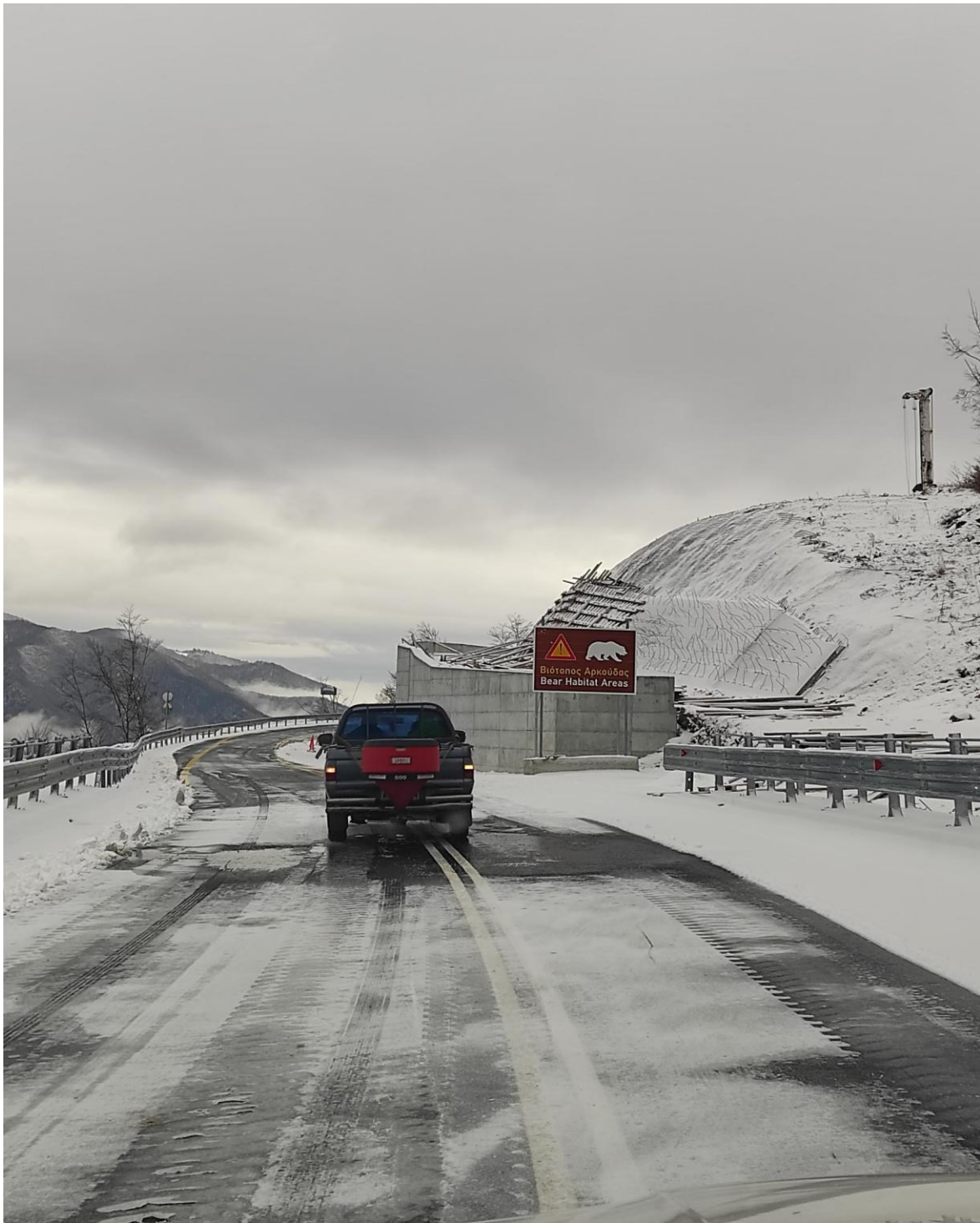
Photo 2: End of the deviation (Cut O20 c.h.. 13+690)
