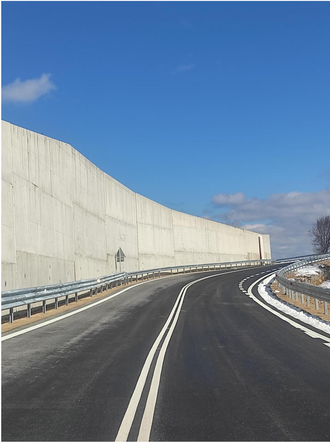
Photo 4: Cut O23 (ch. 14+900)
