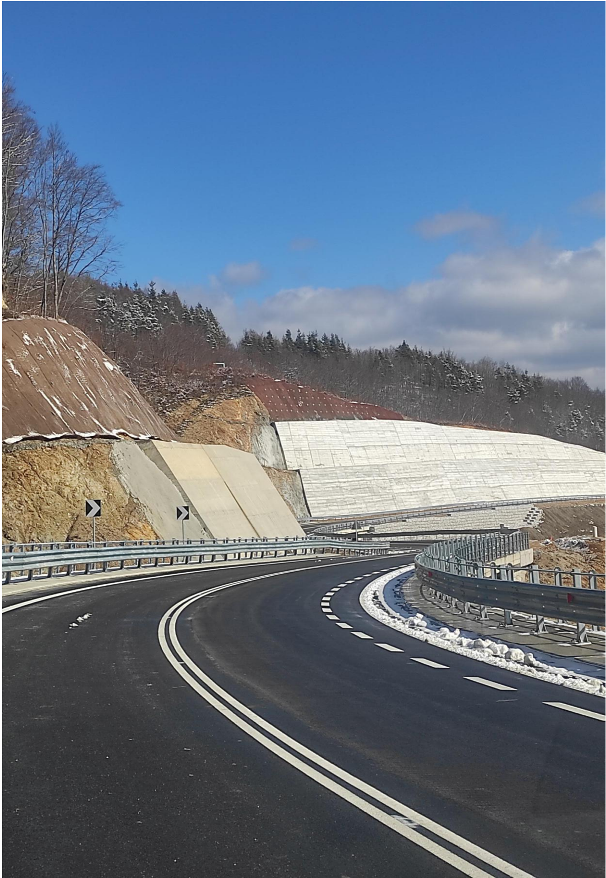
Photo 5: Cut O25 (Ch. 15+600)
